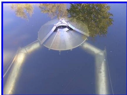
Above: Screen can be adapted to fit on existing intakes in shallow areas or be made retrievable.
