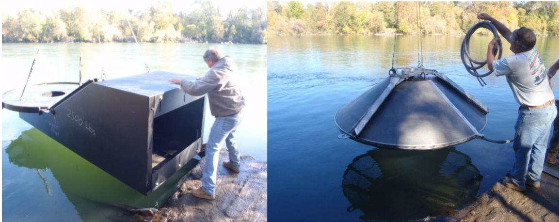
**Figure 1. Installation of a cone screen and its base at Lake California diversion on the Sacramento River. (Photos courtesy of CDFW)**
