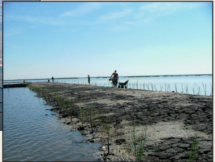
Terrace Planting Crew, Black Lake Terracing Project
